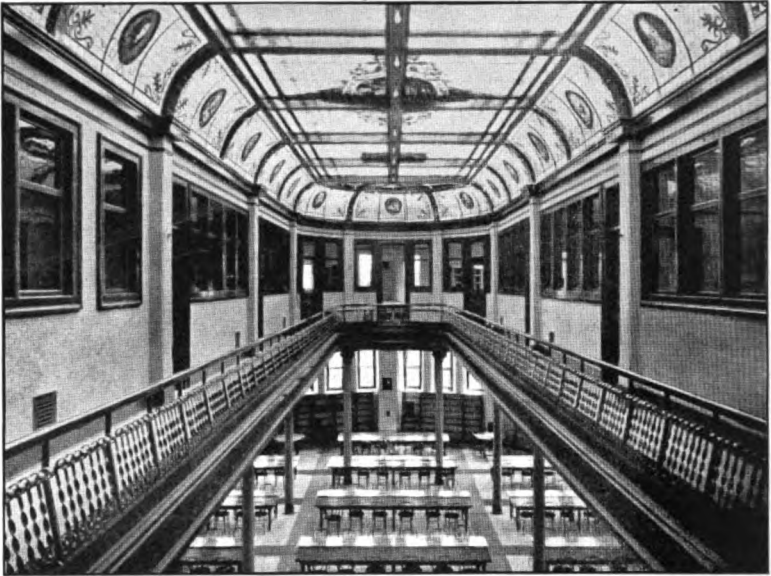
THIRD FLOOR BALCONY AROUND SKYLIGHT OPENING To the Main Reading Room below. Showing Subskylight, Doors and Inner Windows to Seminar Rooms on Sides and End
